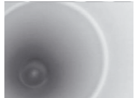
Image 9 Inspection of an AMAXPRO piping at a pipe-to-pipe joint
