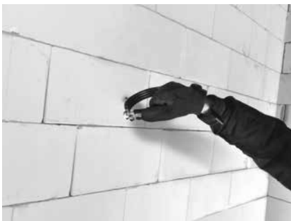
Image 21 Drive the wall plugs into the holes and install each pipe bracket by screwing it into the wall plug.
